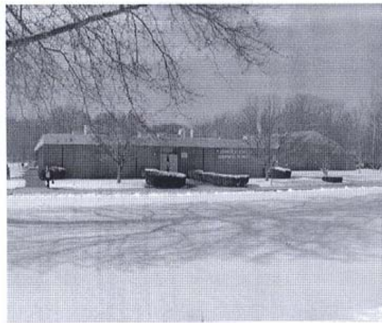
Korn Elementary School
